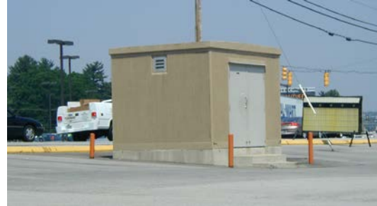
Kmart Pumping Station
