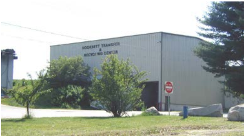
Town of Hooksett Transfer and Recycling Center
