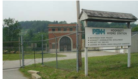
Hooksett Hydro Station
