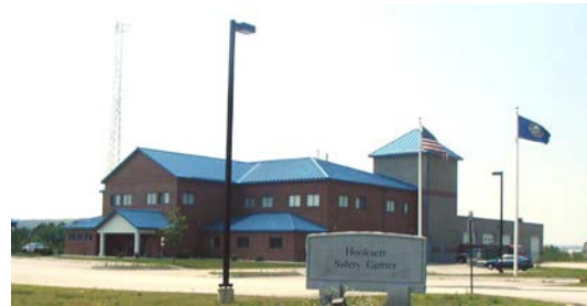
Emergency Operations Center
