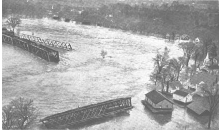
FLOOD SCENE. WRACK AND RUIN AT HOOKSETT, N. H.
